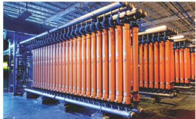
Pall Microza microfiltration membranes provide an absolute barrier to pathogens and remove any particles greater than 0.1 micron that are not removed during sedimentation.
